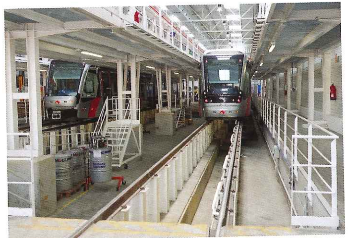
▲ Inspection tracks at Valdespartera depot. There is stabling for 18 trams and it is the main maintenance facility for the system.
